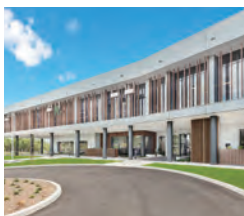
Fujitsu General (Aust.) Pty Ltd. (Australia)
