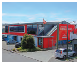
Fujitsu General New Zealand Ltd. (Nowa Zelandia)
